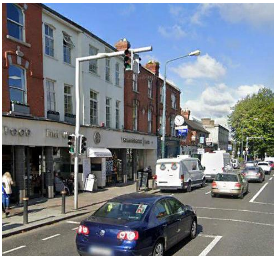
Figure 2-9-12: Example of a gantry traffic signal in Donnybrook (Google Earth)
